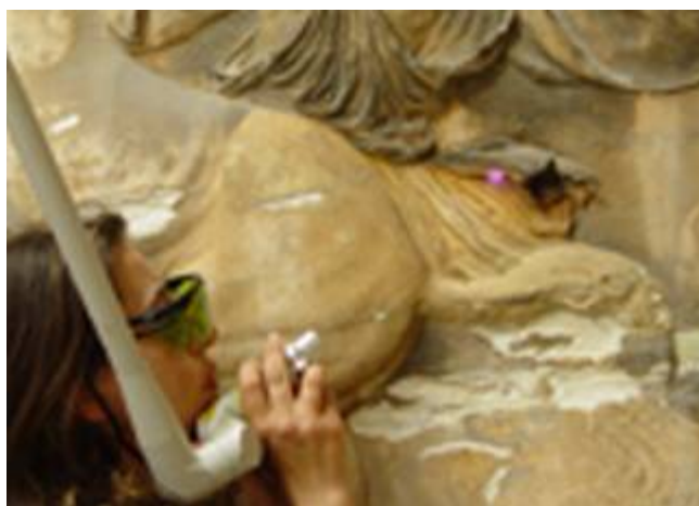
Fig. 10. Laser cleaning of the West Frieze Block - BVIII
