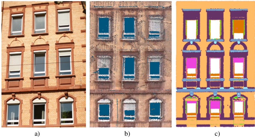
Fig. 1. Results of segmentation: a) façade picture; b) colorized point cloud of the façade; c) segmentation results. Each colour depicts a planar cluster on the façade.
