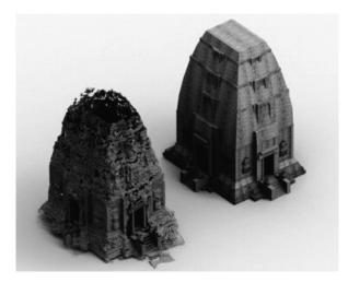
Figure 4: Laser scan and model of Sambor Prei Kuk central shrine.
