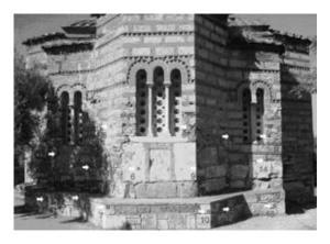
Figure 7: Target positions measured on the façade
