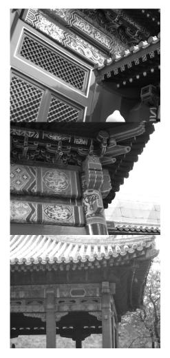
Figure 1. Three photos showing the colour decaying on historical buildings in the Forbidden City, Beijing, China. Top: a recent repainting (presumably with the original colours); middle: colours started to decay; and bottom: significant colour fading.
