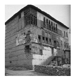
Figure 1: Typical earth –block masonry of the 19<sup>th</sup> cent. in Veroia, Greece (Papayianni, 2006).
