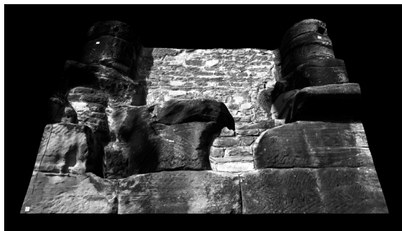
Figure 8: Hybrid data model of parts of the Porta Nigra – 3D laser scanning combined with high resolution images
